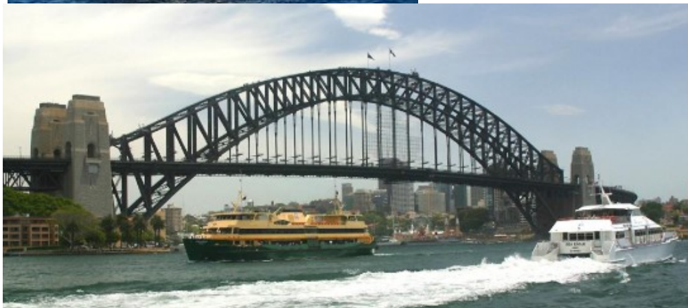
Sydney Harbour Bridge
